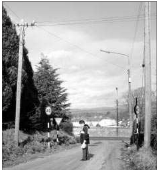
The CHM2000 being used to measure the height of the overhead cable
