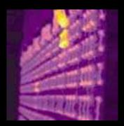
Infrared imaging identifies bad battery cells in an air traffic control emergency backup system, preventing a catastrophic failure.
