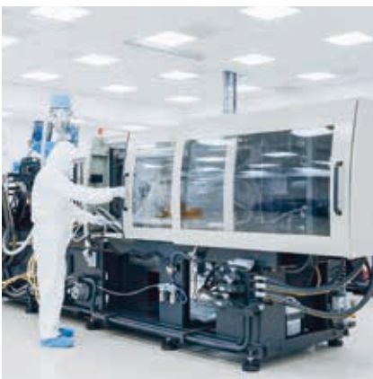
Investigate power supply conditions
