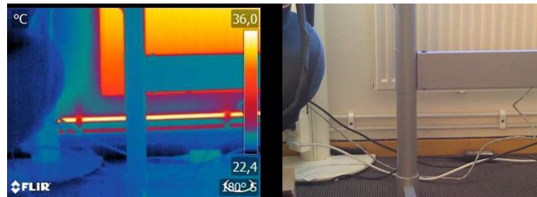
Figure 16.6 “Thermographic inspection” of an inaccessible object.
