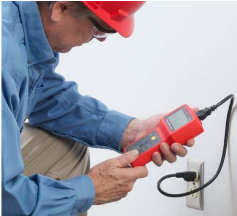
Verify in seconds whether a building's wiring (including voltage drop under load) complies with electrical code.
